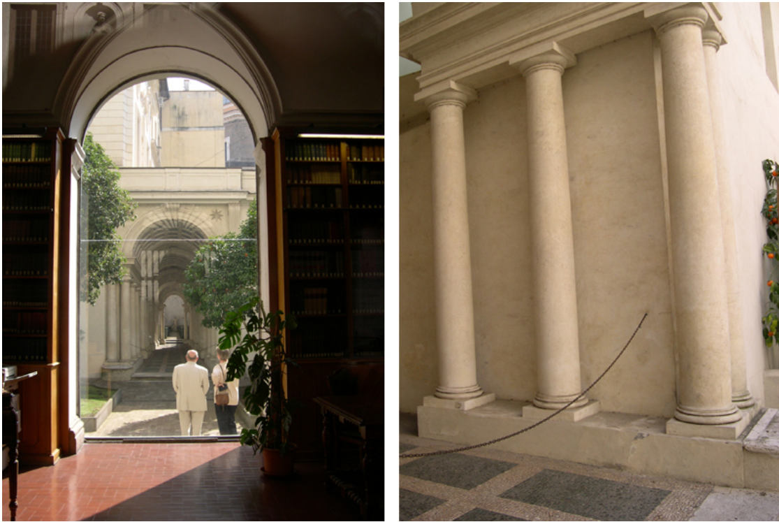
Figure 2.14: Images of the Borromini gallery show the colonnade as seen from the ideal station point ( left ) and from an off-axis view ( right ). Note the warped geometry which creates the illusion of more depth than actually exists in the scene.
